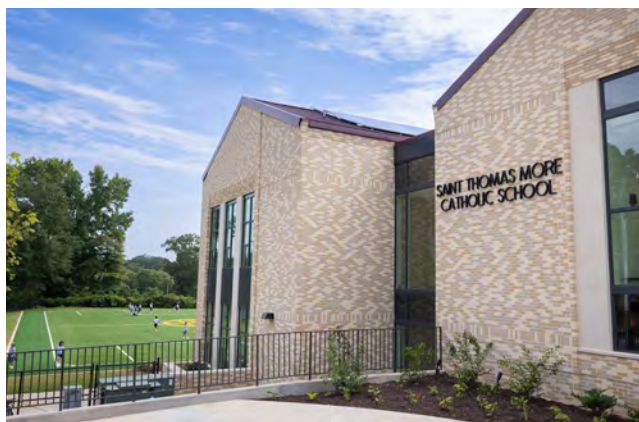
Campus-wide improvements include new K-5 solar-powered classroom building and a new turf field with sustainable drainage system beneath.
